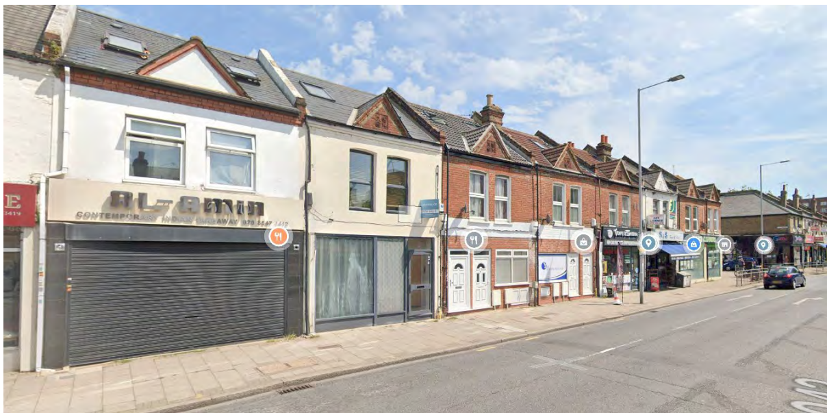
Gloucester Road junction:
